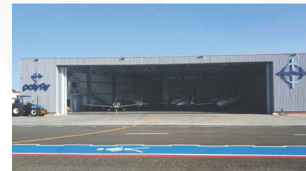
Navegantes, SC – Brazil Hangar PolyFly
