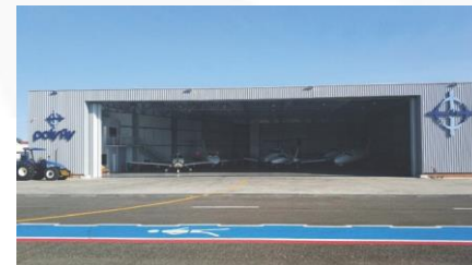
Navegantes, SC – Brazil Hangar PolyFly
