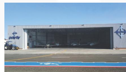
Navegantes, SC – Brazil Hangar PolyFly
