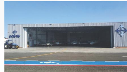
Navegantes, SC – Brazil Hangar PolyFly
