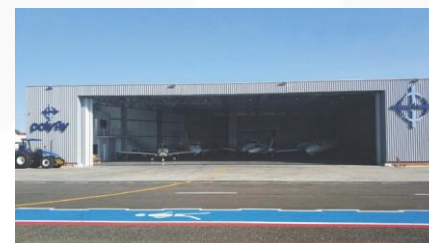
Navegantes, SC – Brazil Hangar PolyFly
