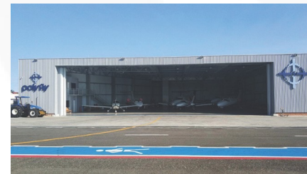
Navegantes, SC – Brazil Hangar PolyFly
