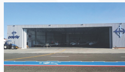
Navegantes, SC – Brazil Hangar PolyFly
