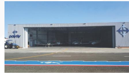
Navegantes, SC – Brazil Hangar PolyFly
