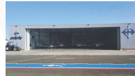
Navegantes, SC – Brazil Hangar PolyFly
