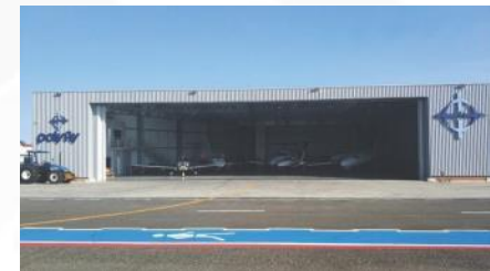
Navegantes, SC – Brazil Hangar PolyFly
