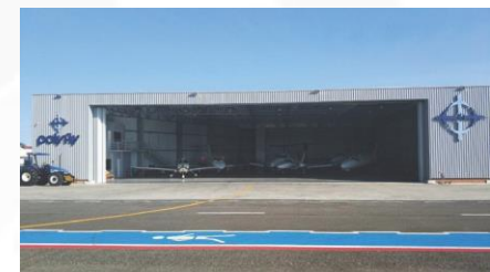
Navegantes, SC – Brazil Hangar PolyFly
