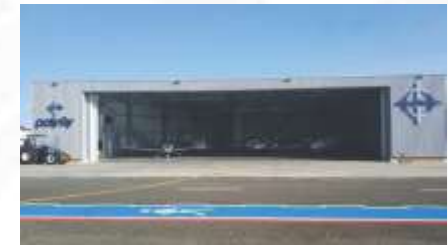
Navegantes, SC – Brazil Hangar PolyFly
