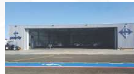
Navegantes, SC – Brazil Hangar PolyFly
